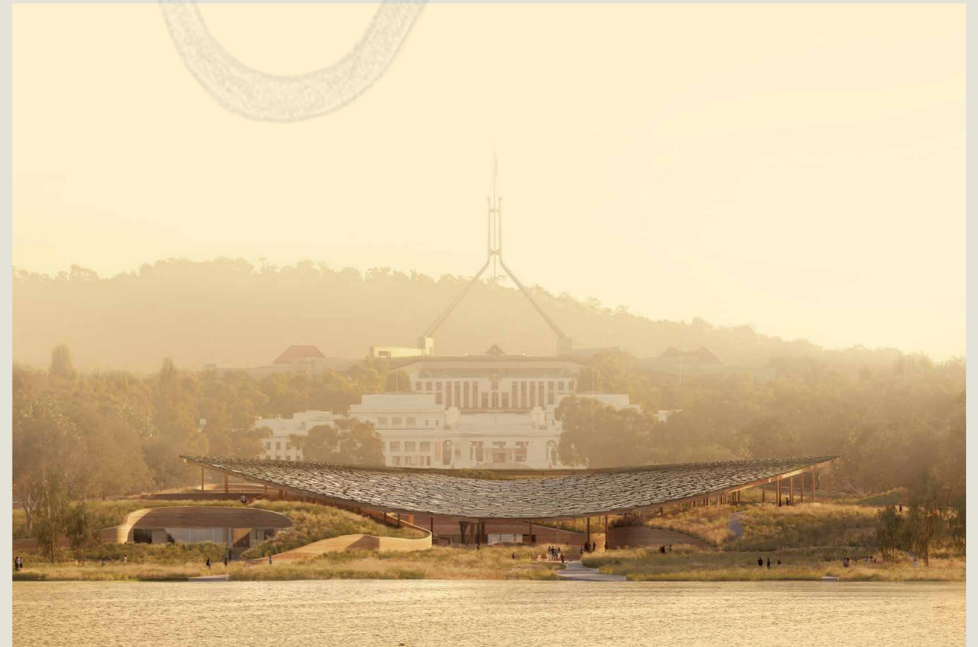
Taking residence within Australia's Parliamentary triangle, in the foreground of Parliament House. Its organic, fluid and curved structure offers a counterpoint to the surrounding colonial structures.
